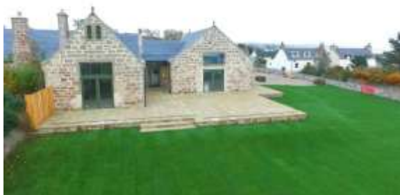
The Old School Embo – post construction
